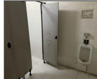
Photo of the sanitary facilities toilet.JPG
