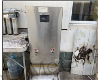
Photo of non-conformity NC-no high temperature warning.JPG
