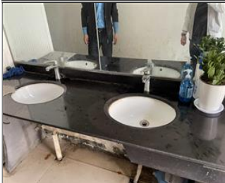
Photo of the sanitary facilities wash basin.JPG
