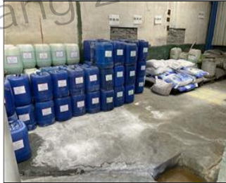
Photo of chemical storage room (if applicable) chemical room.JPG
